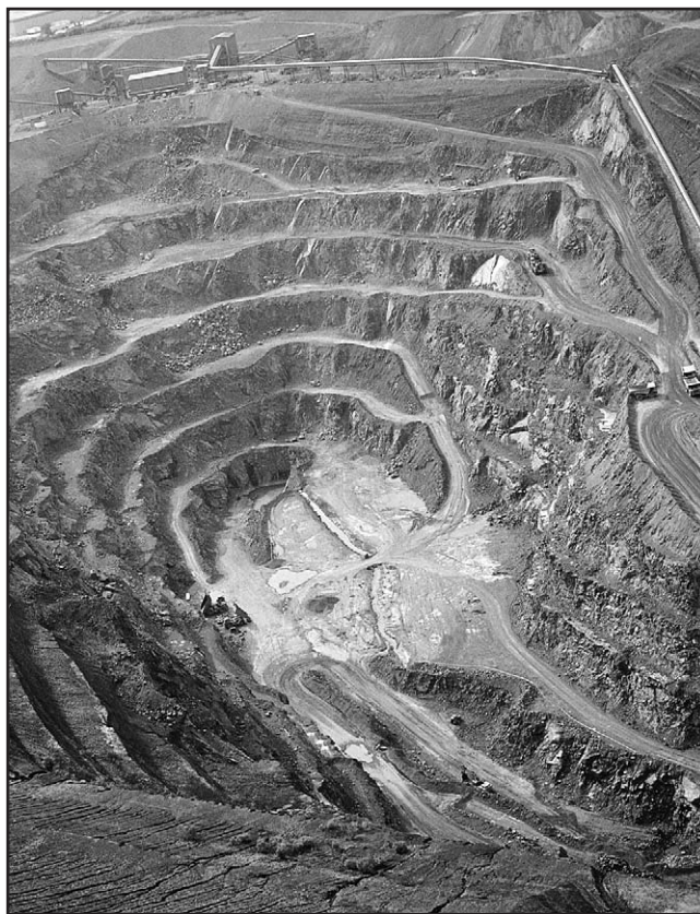
Aerial view of Cliffe Hill New Quarry, working South Leicestershire Diorite. (Photo: Tim Cullen, BGS © NERC)
